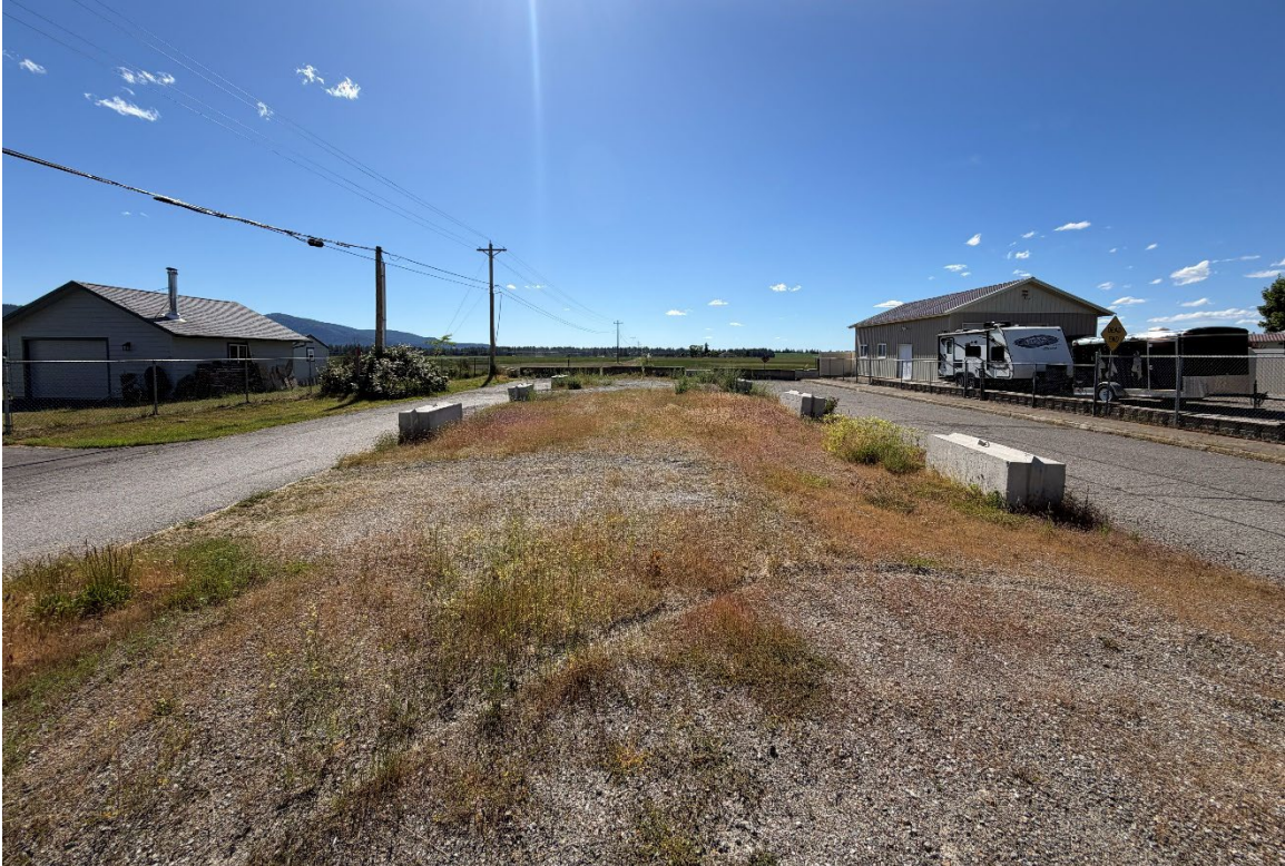
W. Nez Perce Rd. Looking west into subject property:
